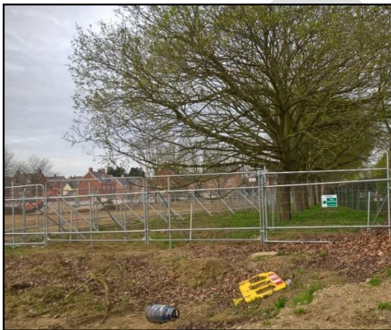
Tree protection at housing site
