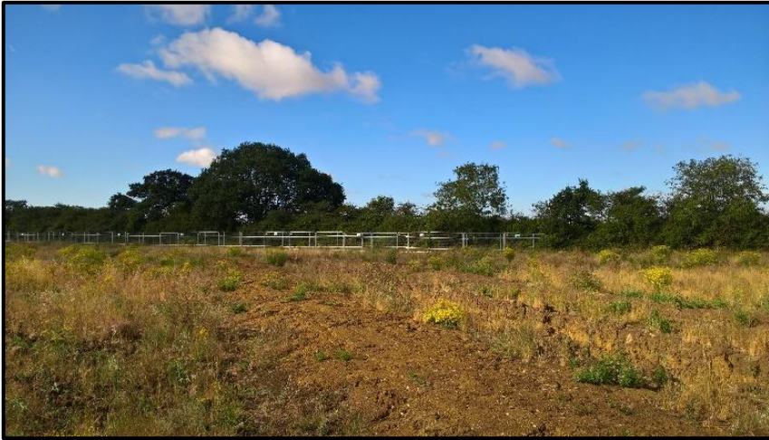
Tree protection fencing in housing construction site.
