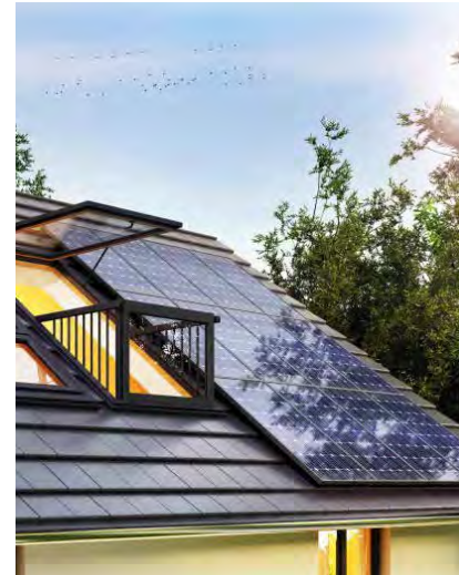
SU.02. Energy efficiency and energy generation
