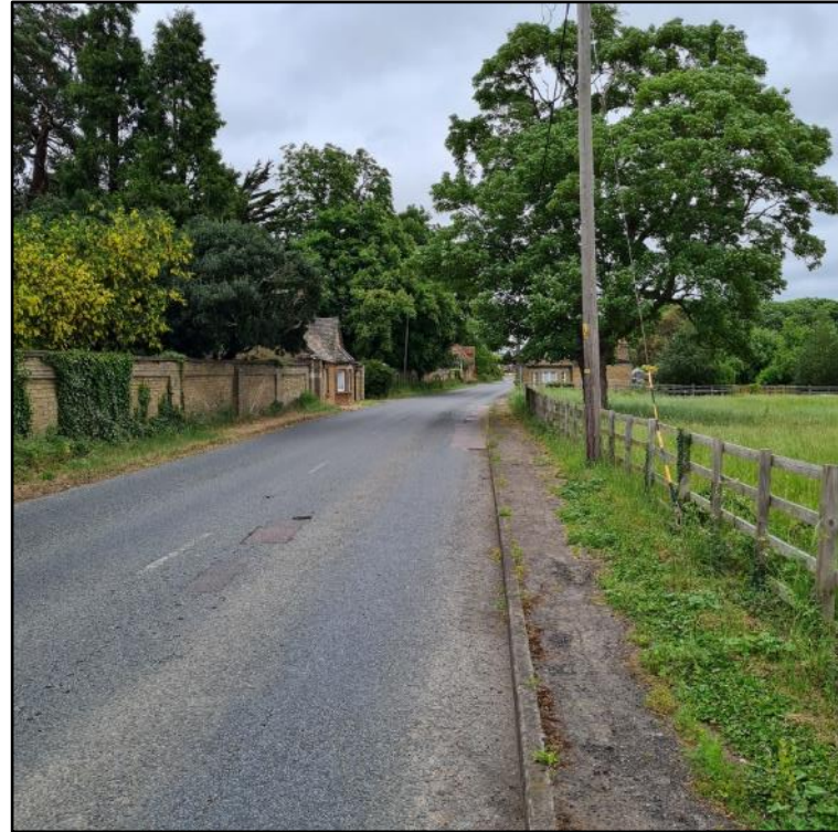
View 2 – Chanelled view north along Barford Road, taking in The Bungalows, boundary wall and South Lodge with specimen trees.
