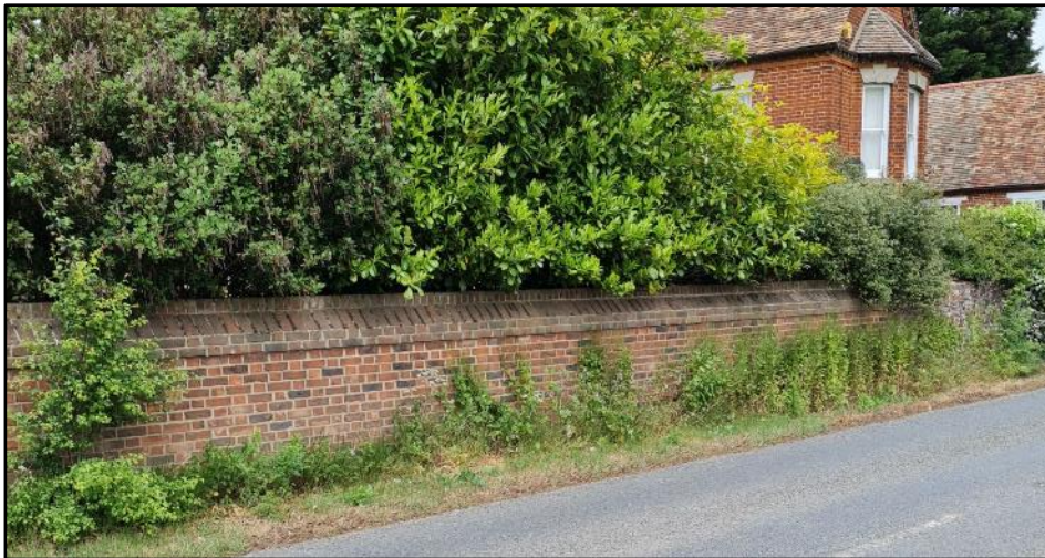
Figure 25 The red brick boundary wall at Lower Farmhouse, which forms one of several walls continuously fronting the west side of Barford Road in the village.
