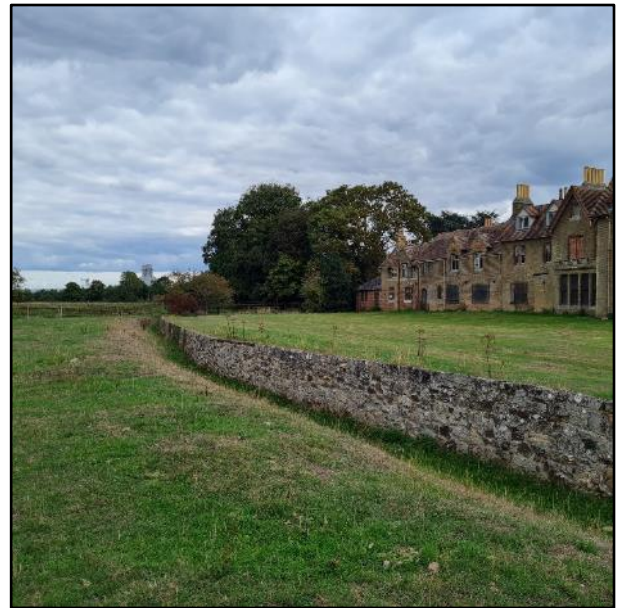
Figure 10 The ha-ha wall to the north west of the New Manor House, designed to facilitate views towards the parkland and possibly the church and 18 th century manor beyond.
