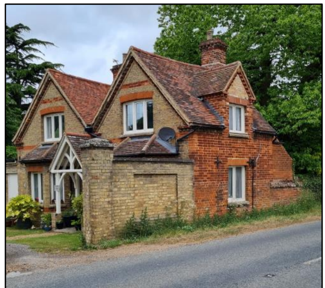
Figure 15 [Above] North Lodge is built from both red and buff brick. The red brick utilised for the east elevation harmonises with the red brick boundary wall which continues northward.
