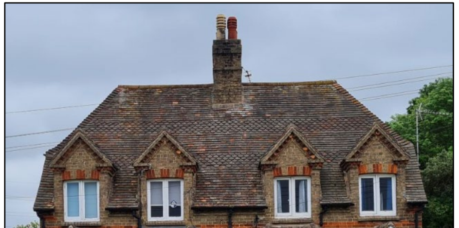
Figure 24 Fishscale tiles used at 1 and 2 The Cottages.
