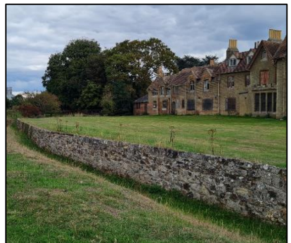
Figure 26 The ha-ha wall running to the west of New Manor House.
