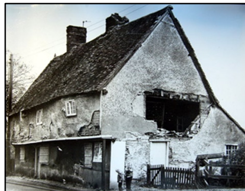
Figure 5 A photo taken of Rowe's Cottages shortly before it was dismantled (source: Historic England).
