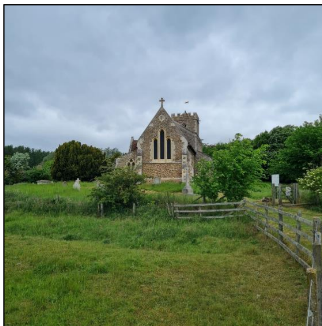
Figure 3 View of St Denys' Church from the east. The ditch in the foreground may point to an earlier use of the site.
