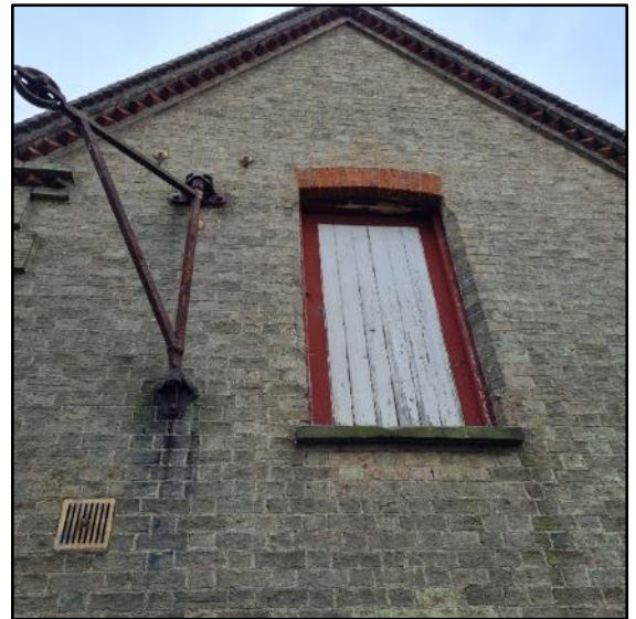
Figure 27 A winch and hayloft at the stables. Where buildings have fallen out of use, historic features have often survived intact.
