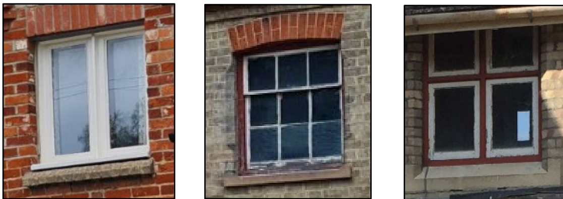
Figure 22 A selection of timber windows to 19 th century buildings in the village - note the red frames to the windows in centre and right-hand images.
