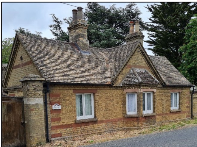
Figure 20 The principal elevation of South Lodge, with dressed stone detailing and a dentil course to the eaves and verges.
