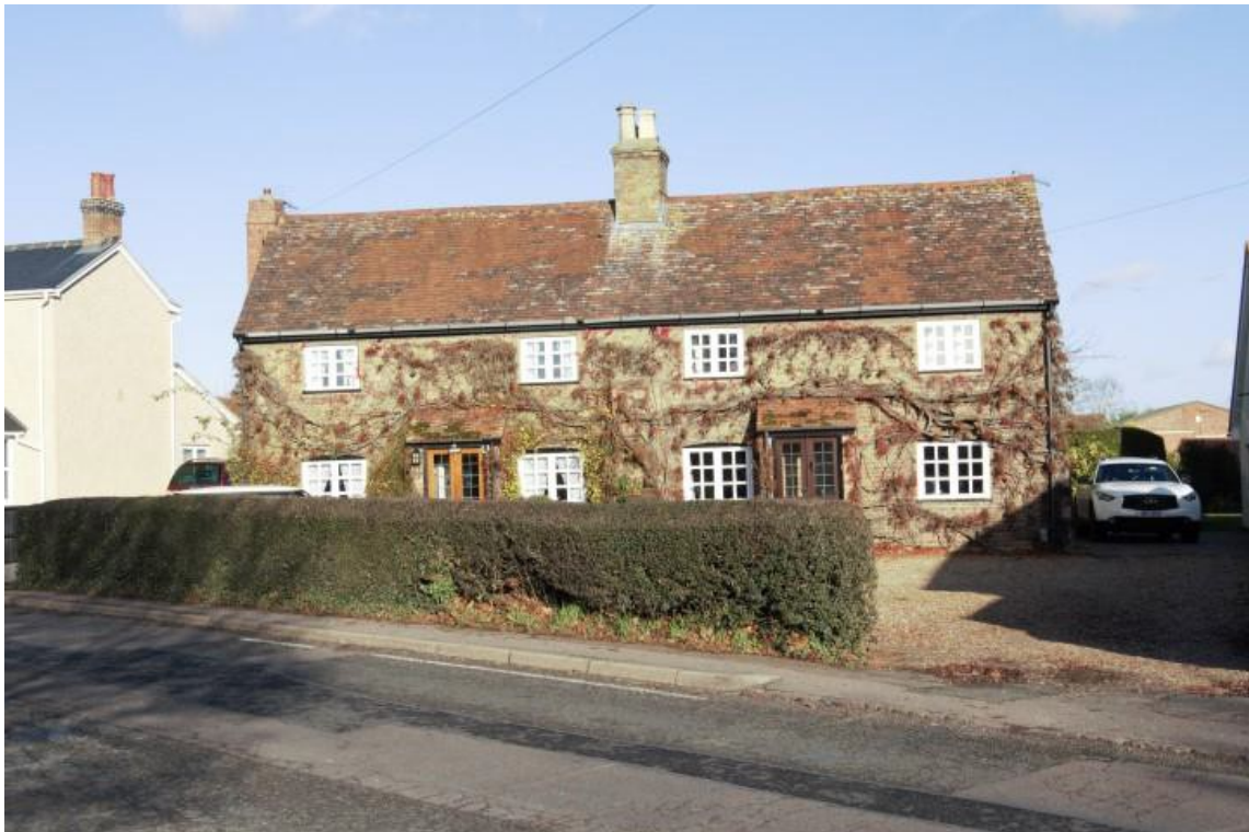
Plate 32 A pair of houses displaying the scale and articulation of much of the traditional property in the village, these featuring a symmetrical facade and axial stacks (though it appears one has been removed since construction).
