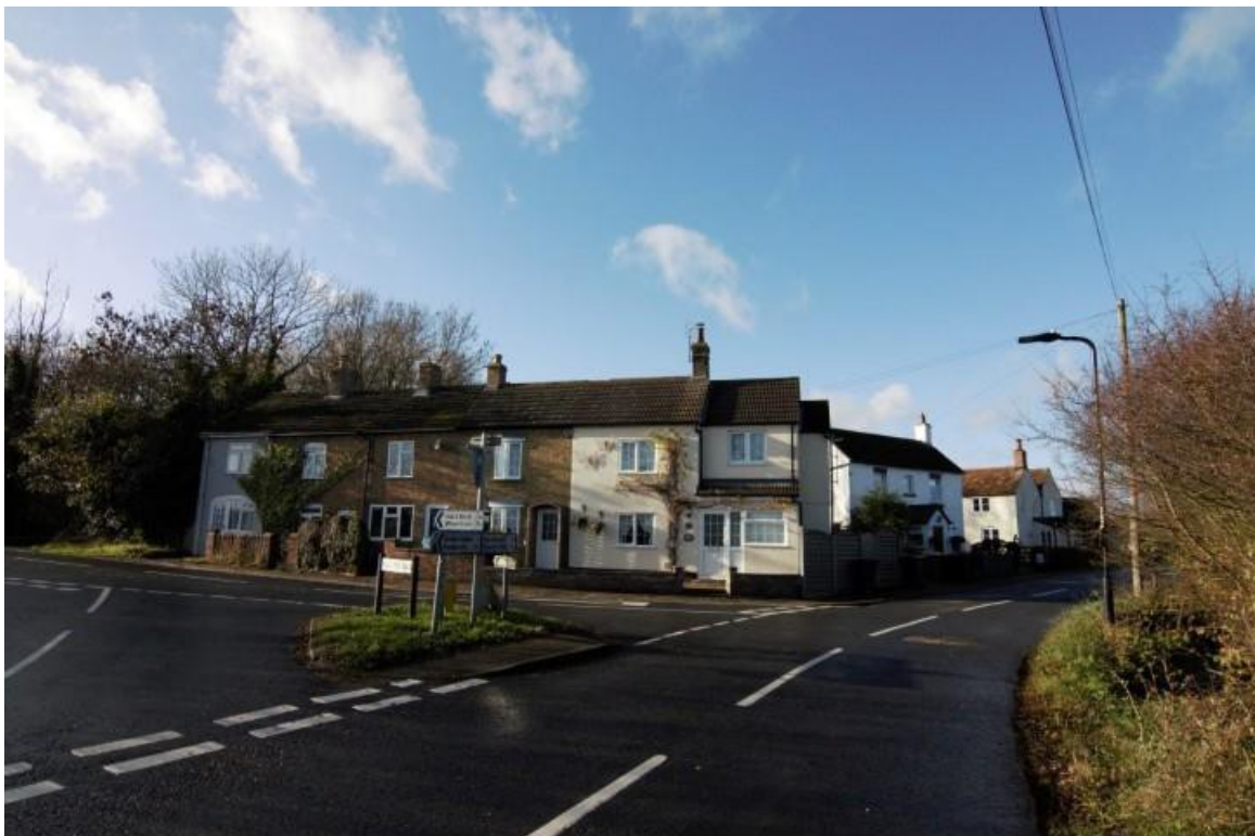
Plate 27 The view south west from Keeley Lane describes a cluster of little cottages hard against the road.
