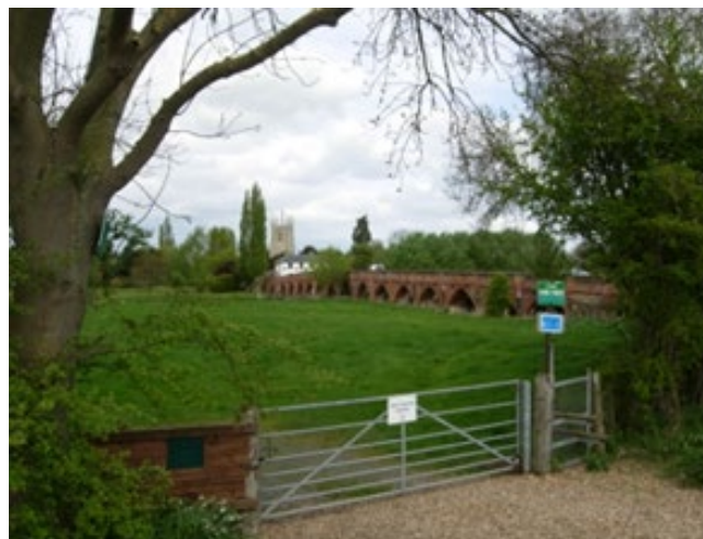
Barford Bridge and Causeway
