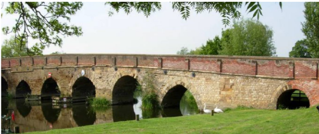
Barford Bridge - Scheduled Monument and Grade I Listed
