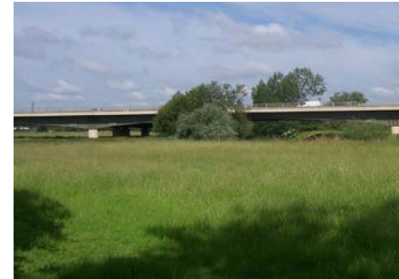
Wildlife can pass beneath the viaduct that carries the A421 Bedford bypass if suitable habitat is created on each flank
