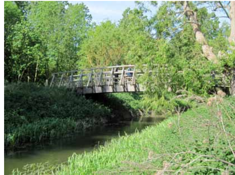
New bridge taking cycle path over Elstow Brook on the Grange Estate
