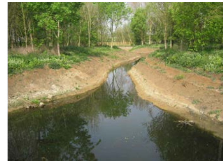
Recently completed river backwaters on the Grange Estate
