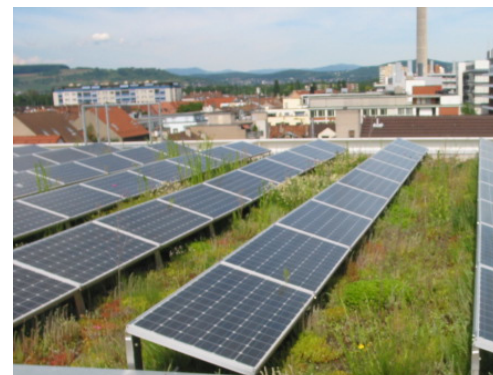
PVs combined with green roofs as seen here in Basel, Switzerland
