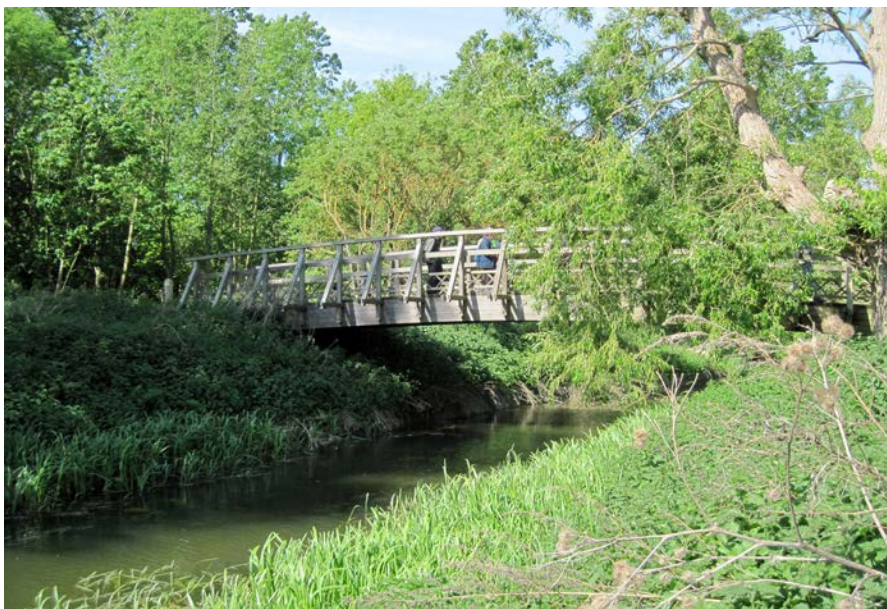
New bridge taking multi-user path over Elstow Brook on the Grange Estate
