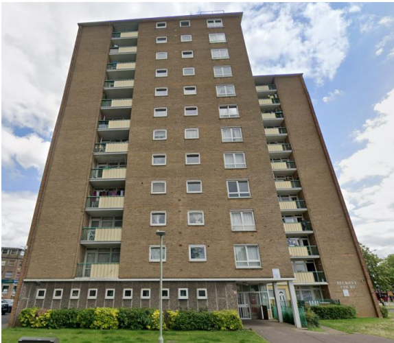
Image 3: Greyfriars block from ground level.
