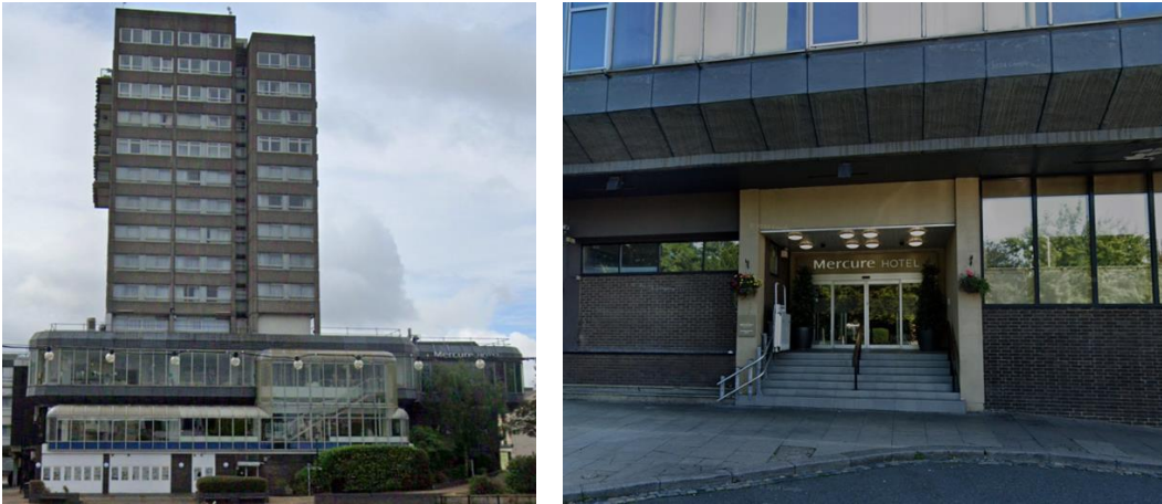
Image 17: North elevation of the Mercure hotel. Hotel entrance
