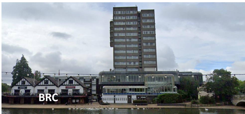
Image 19: View looking south of the Mercure from the north bank of the River Great Ouse showing built heritage context
