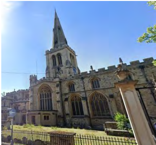
St Paul's Square, Town centre Image source: Google maps
