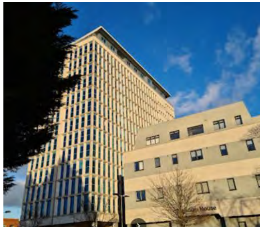
Meridian House off Kingsway Link Image source: Google maps
