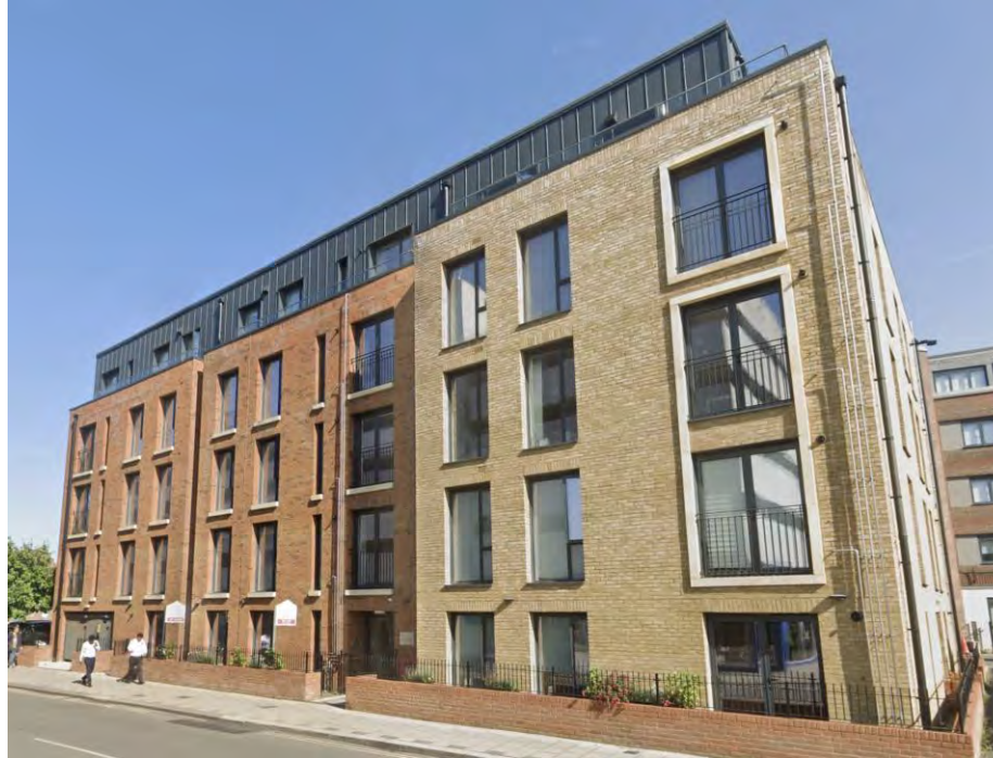
Lurke Street apartments
