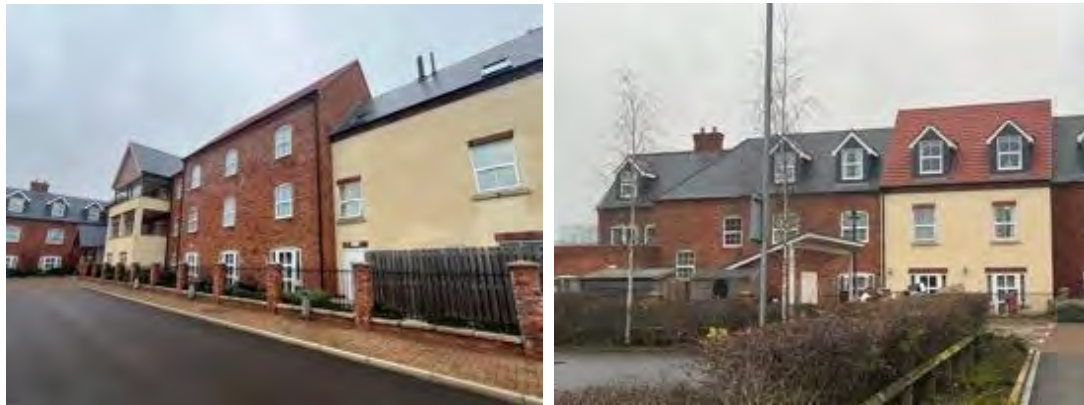
Building composition lacks harmony, especially in terms of overall massing, roofline and materials palette
