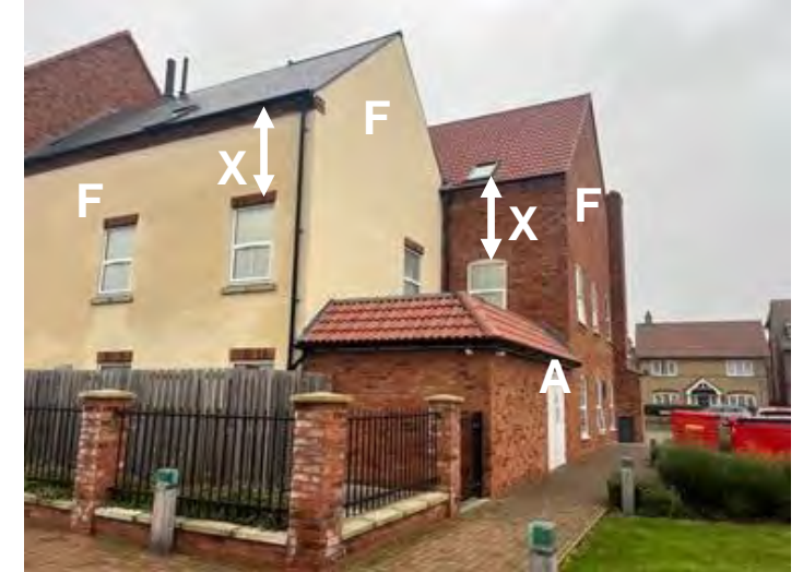
Poor massing and location of ancillary room at 'A'.
