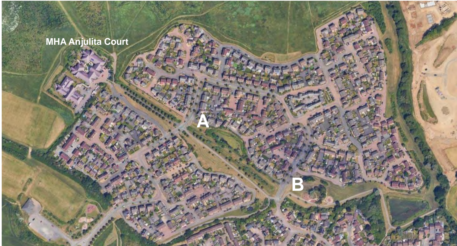
Woodlands Park/Ashmead Road showing dominant green infrastructure through the site.
