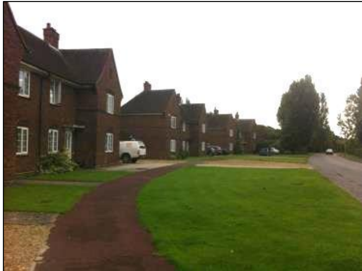
Fig. 24. Green Lane, looking west
