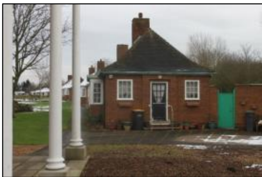
Figs 80 & 81. 1964 phase of development, end elevation with square windows (left), block-like chimneys with copper flashing (right)
