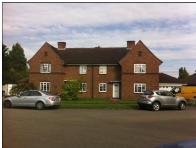
Fig. 25. Churchill Close, gable ended house type
