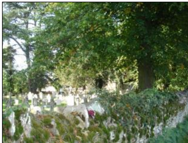
Fig. 28. Stone walls of St James's church yard
