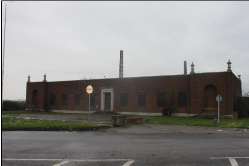
Fig. 31. London Brick Company Headquarters, south elevation
