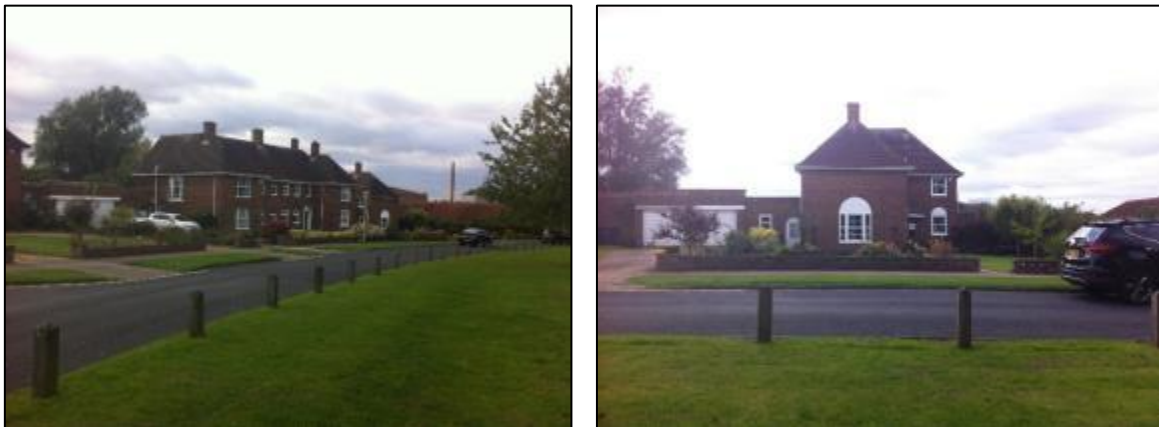
Figs. 40 & 41. Large houses on The Crescent (left), detached end house (right)
