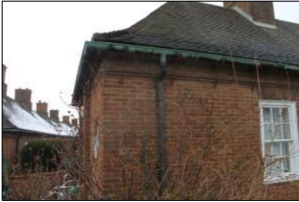
Figs. 66 & 67. 1956 phase of development showing copper guttering (left) and bay window (right)
