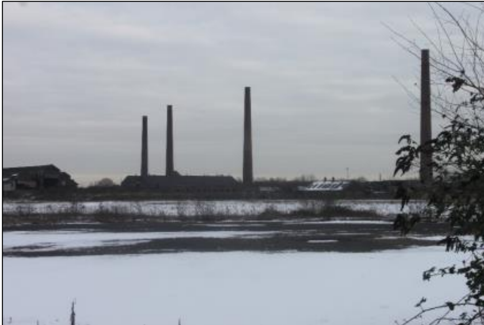
Fig. 2. Stewartby, view from west of listed chimneys and kilns
