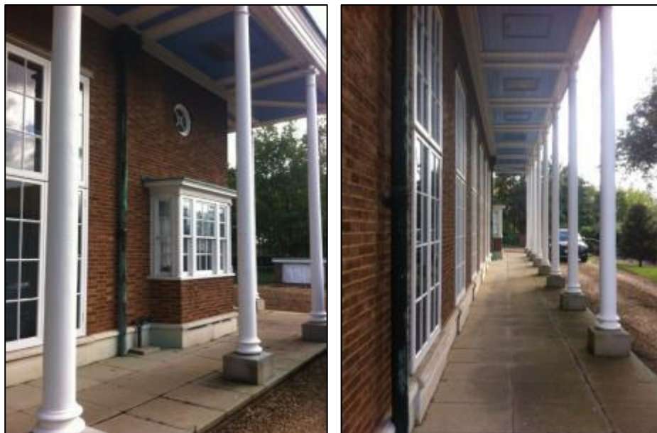
Figs. 76 & 77. Common Room, west elevation, bay window and downpipe (left) and coffering (right)
