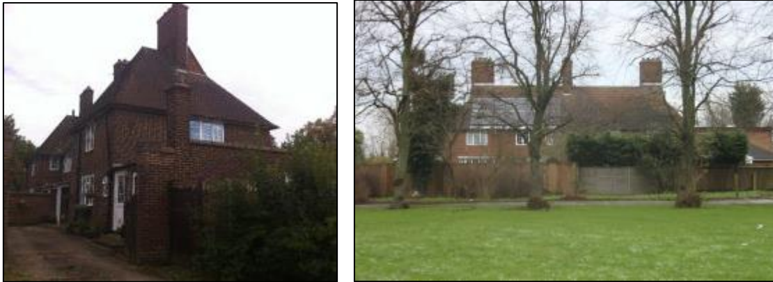
Figs. 34 & 35. Pillinge House and Broadmead House, west elevation (left) and south elevation (right)
