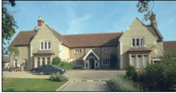
Fig. 6. Manor Farm House (now hospital)
