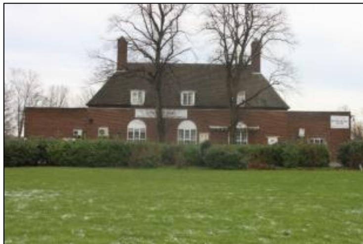
Fig. 36. Club House, west elevation
